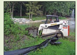
Backfilling Soil
